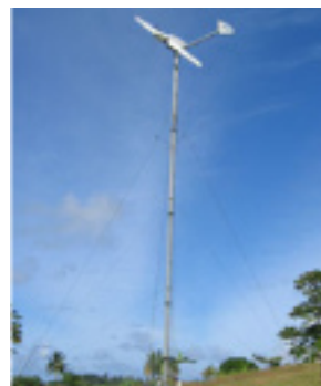
Wind turbine in Fiji. Photo courtesy of UNEP Risoe Centre
